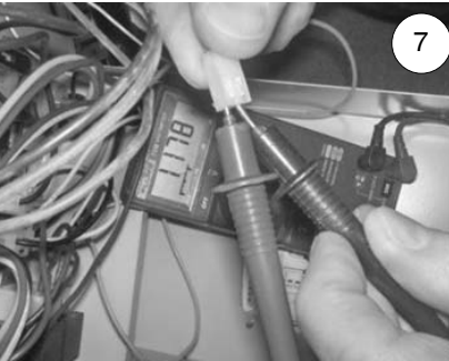
7 Measuring upper sensor resistance through wire harness (disconnected at control board).
